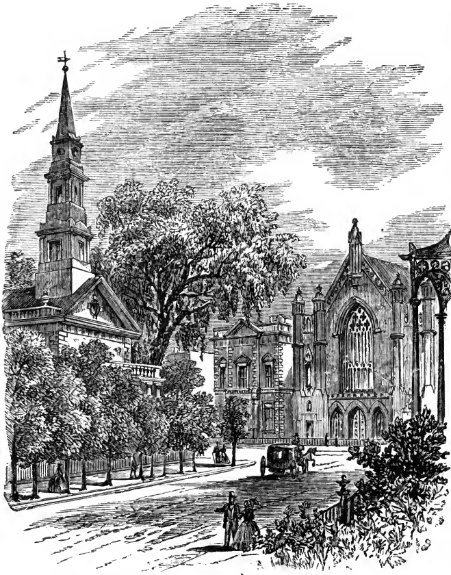
HISTORICAL SOCIETY BUILDING AND ST. MARK'S CHURCH.
